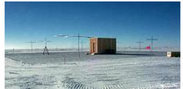
Meteor radar station on the South Pole
