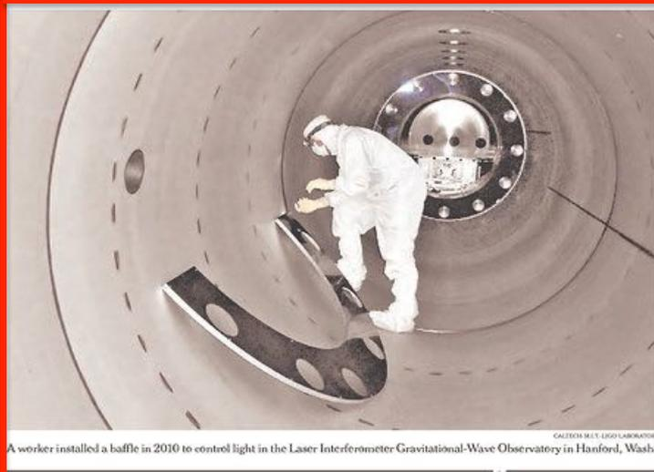
A worker installed a baffle in 2010 to control light in the Laser Interferometer Gravitational-Wave Observatory in Hanford, Wash.
